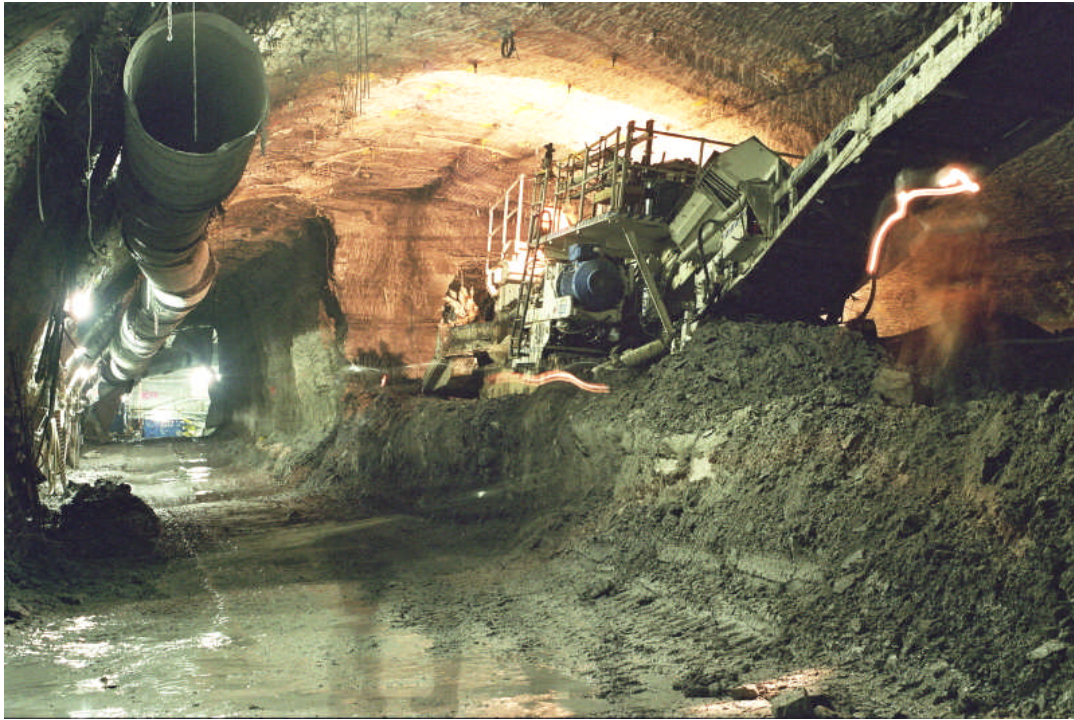
Photograph 2. Macquarie Park Station – Platform Cavern, top heading
