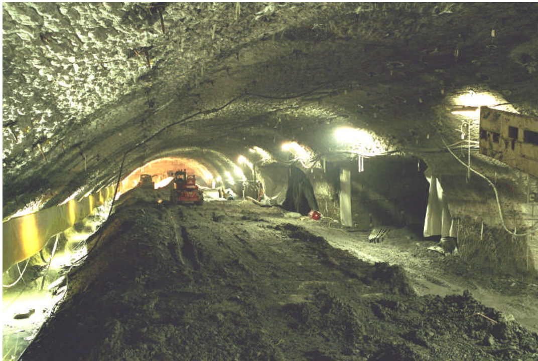
Photograph 1. Macquarie Park Station – Platform Cavern, top heading
